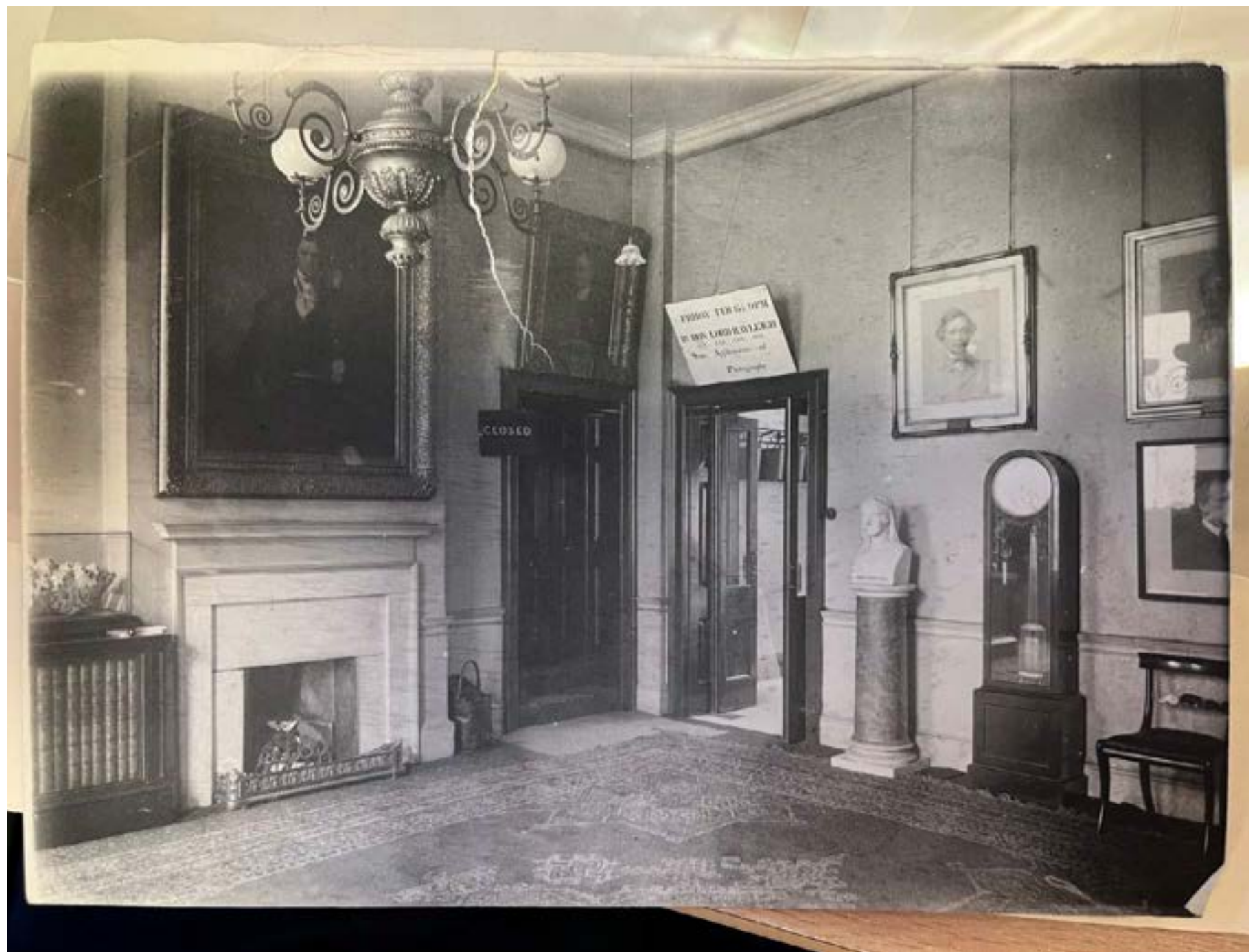
Fig 3.125 Mid-1890s Katherine M Reynold's photograph of the north-east corner of the first-floor Ante-Room. Note the handsome (probably mahogany) doors and doorcases, the steps up into the Theatre and the relative simplicity of the cornice and the fire surround. Ri Archival Collection – Reynolds Collection
