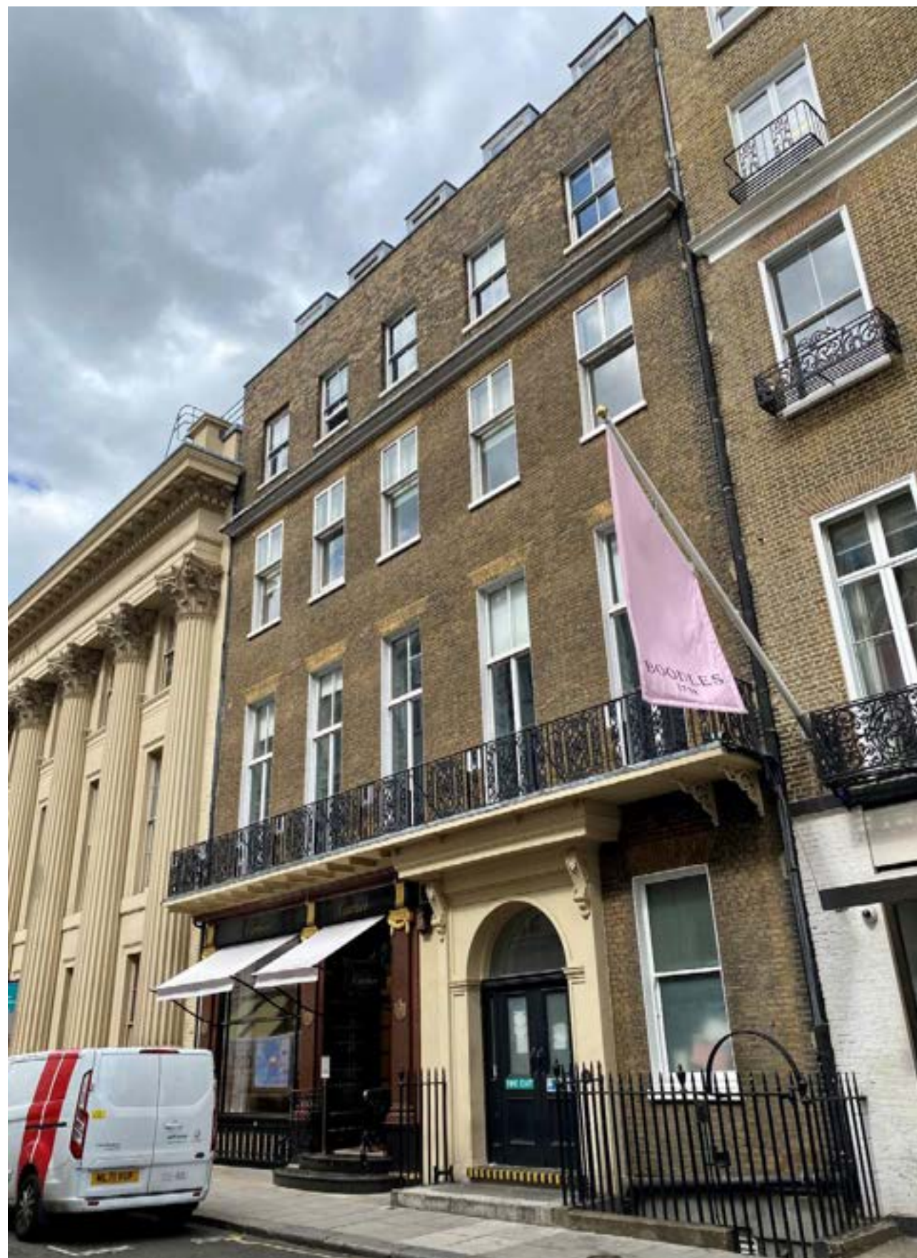
Fig 3.103 No 20's shopfront was installed between the wars when the ground floor was first leased to Cartier
