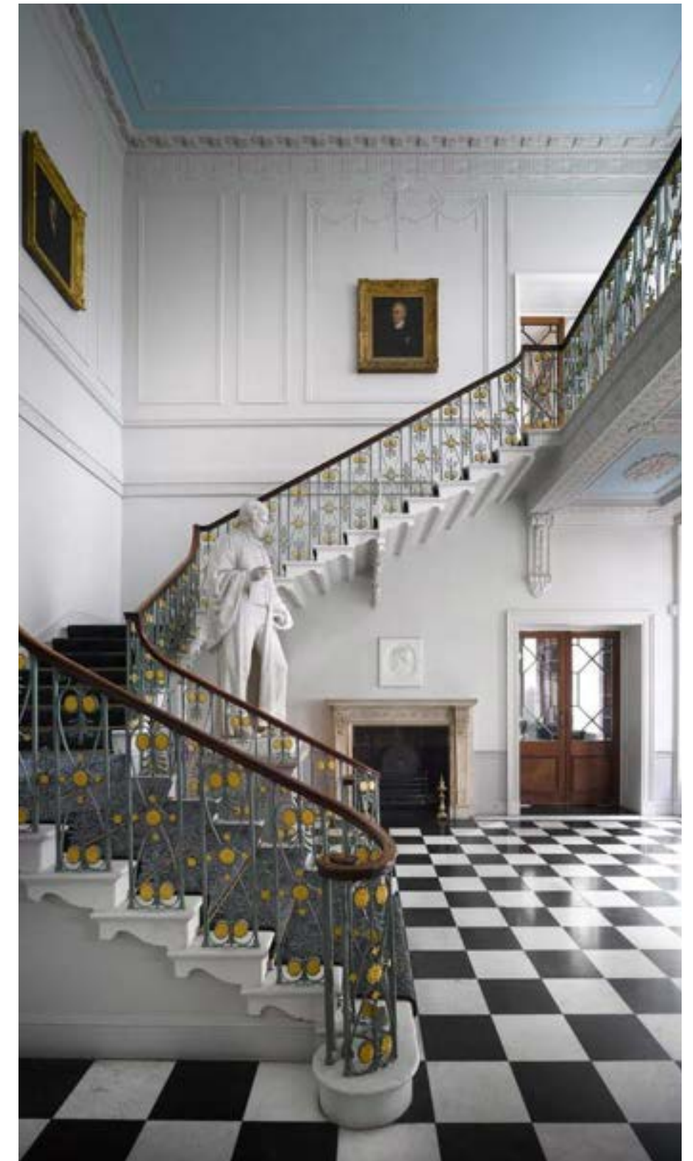
Fig 3.124 The Grand Stair Hall's unapologetic black and white marble floor was an early 1930s LR Guthrie introduction. At this date the original floor was removed for replacement with one of reinforced concrete. The half round headed opening in the wall at the head of the stair's first flight was introduced in the first decade of this century, as part of the endeavour to make the Ri more inviting, open and accessible
