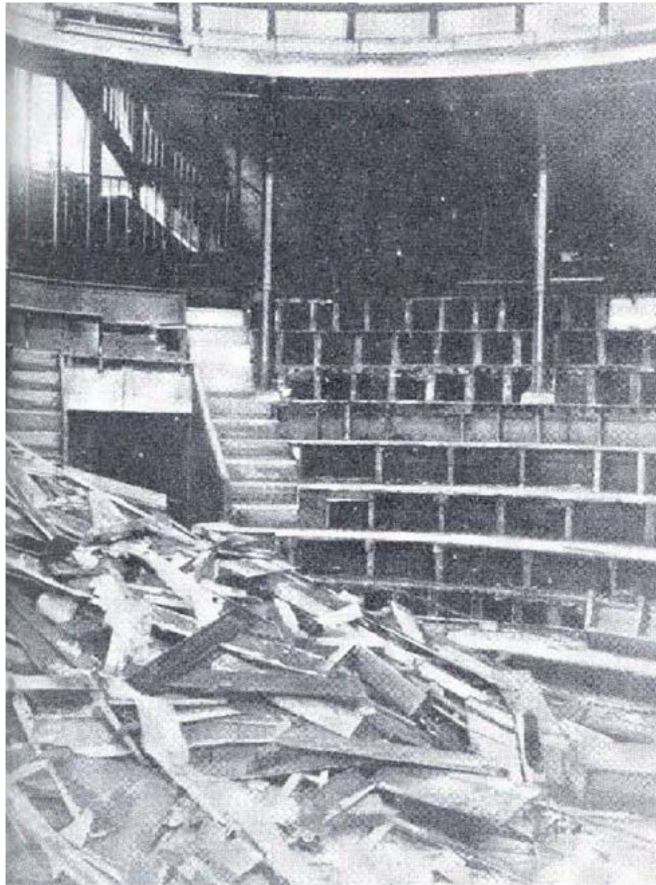
Fig 3.104 Demolition of Lecture Theatre. WJ Green, 1929 photograph, from Proc.Roy.Inst. , 1956, 36, 543-67, facing p. 556
