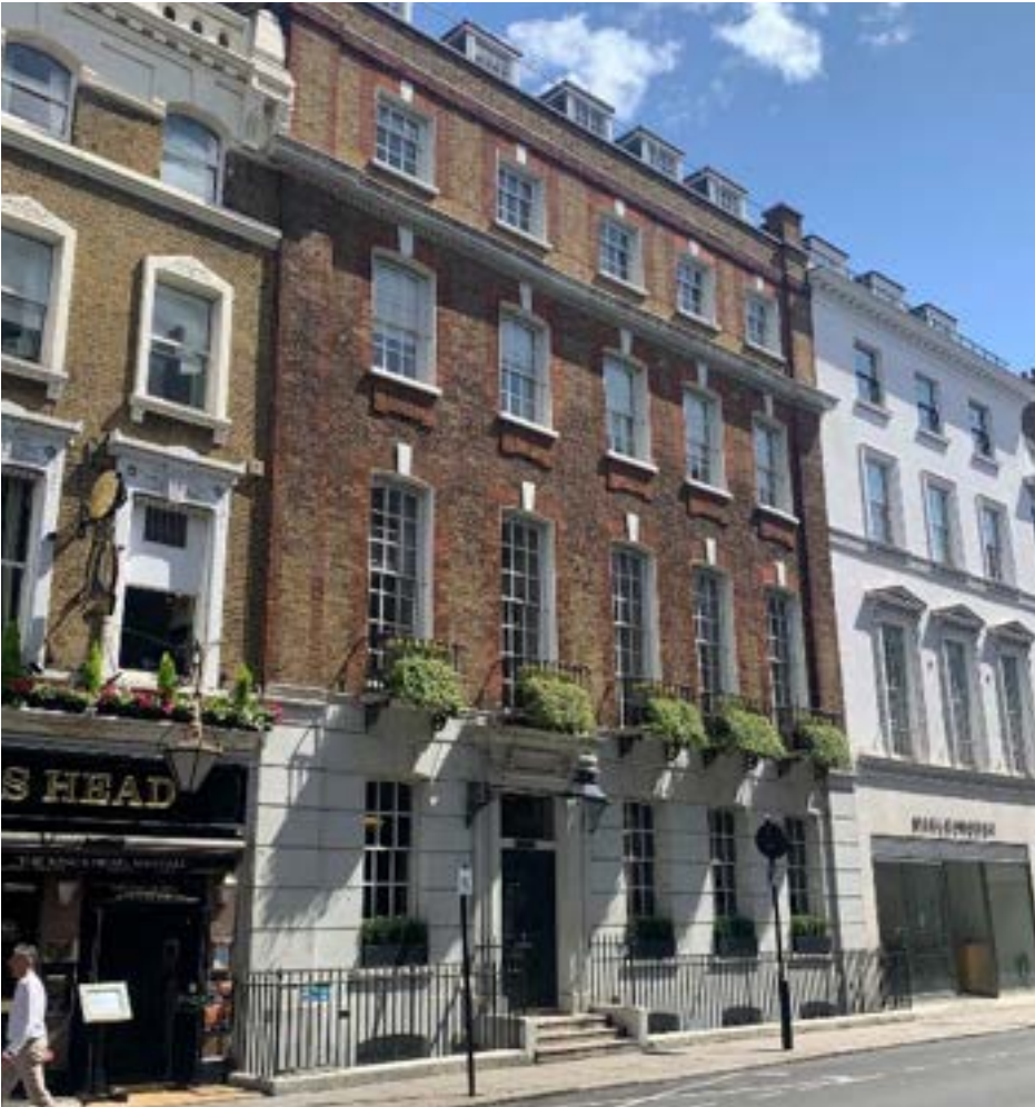
Fig 3.58 7 Albemarle Street showing earlier facade
