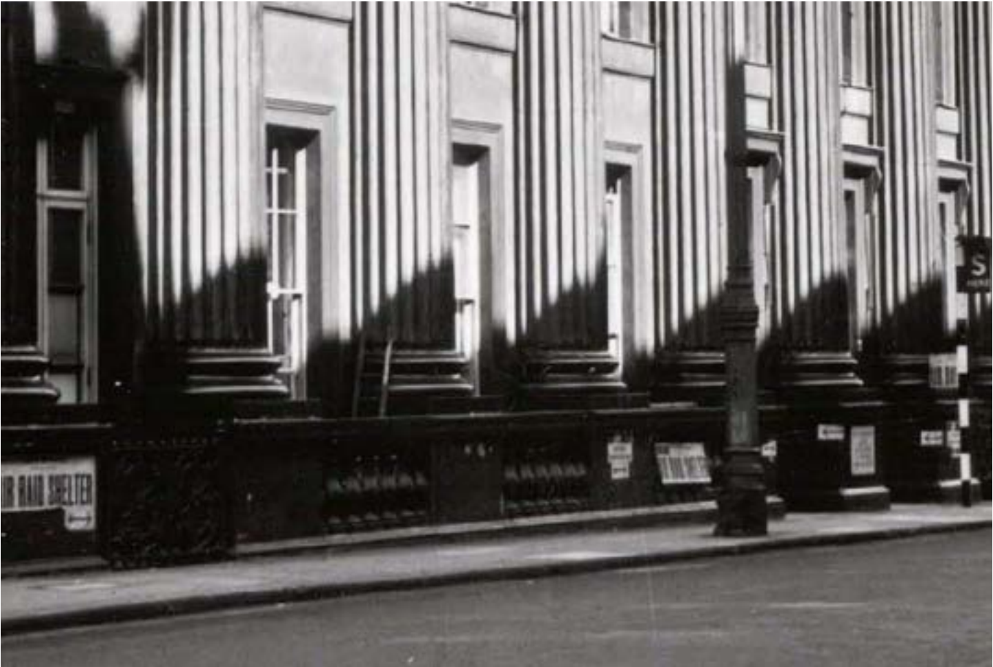
Fig 3.128 Detail of a photograph showing the Ri in 1941 when it housed an air raid shelter, NMR BB032583
