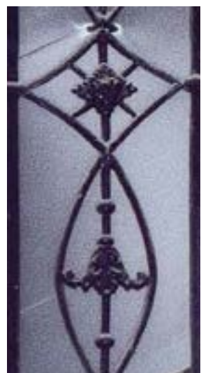
Fig 3.66 Detail from No 20's staircase
