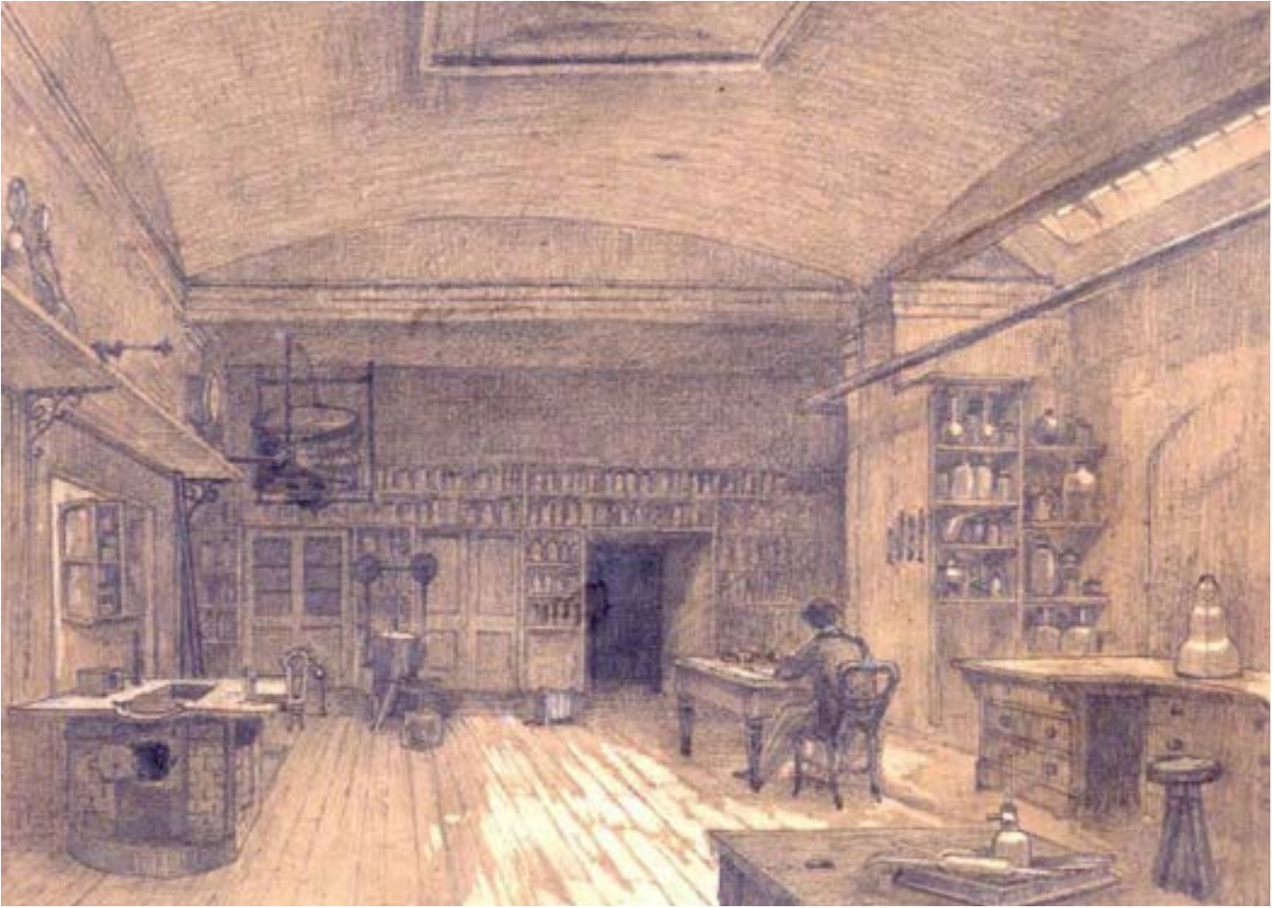
Fig 3.91 Interior of old Eastern Laboratory before demolition. Charles W Dempsey, pencil drawing, summer 1872, RIIC 0452
