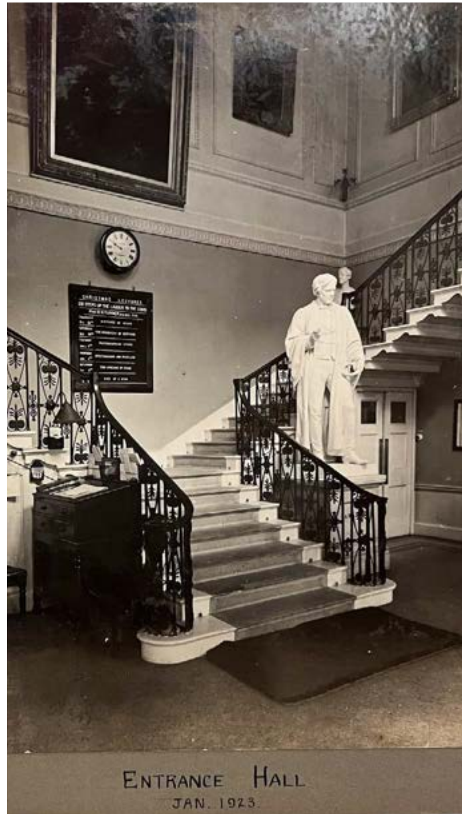
Fig 3.123 Taken in January 1923, this photograph provides an invaluable record of the Grand Stair Hall's form prior to the transformative works of the early 1930s. Note the wall mounted clock and noticeboard at the head of the first flight of stairs, the portraits cutting across the primary plaster frames, the corner fixed lighting arrangement, the under-stair door and the plain flooring. Ri Archival Collection
