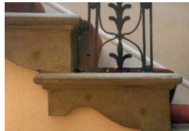
Fig 3.65 Section of step at Basildon Park
