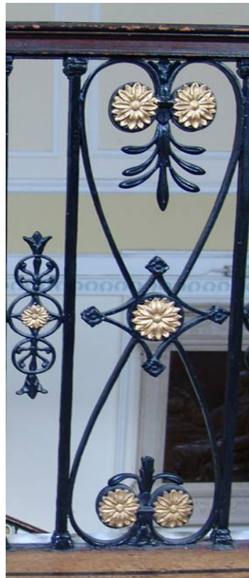
Detail of staircase banister.
