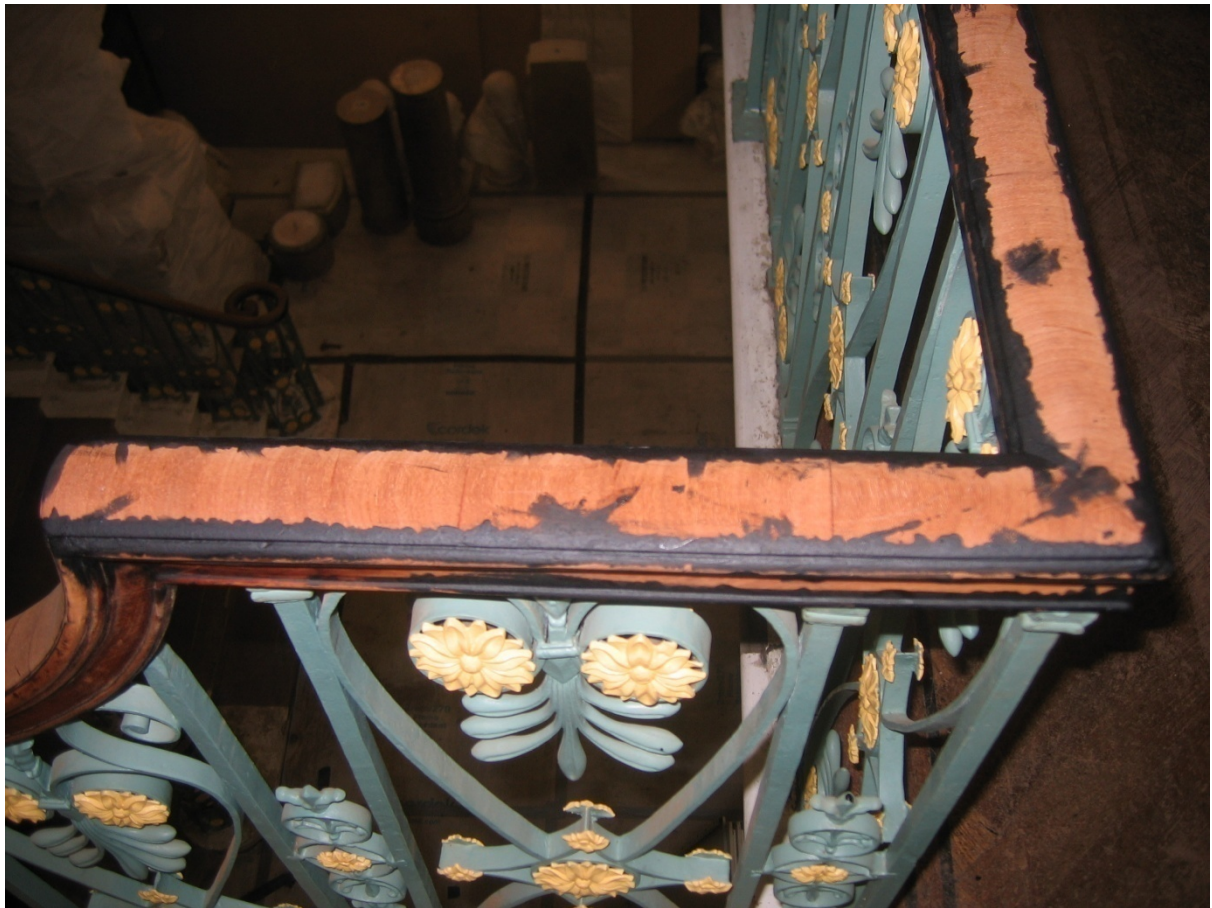
The wooden handrail back in place on the conserved metal banister.
