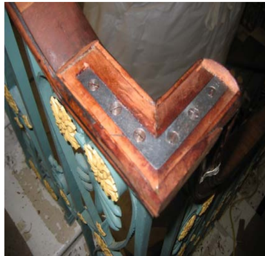
Reinforced corner to provide structural stability.
